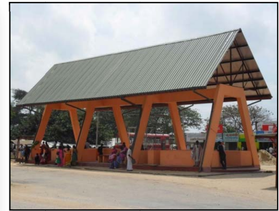
Chavakachcheri Bus Stand was constructed at a cost of Rs. 4.0 Mn
