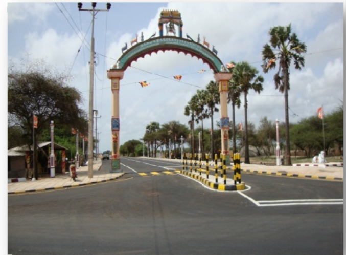
Thiruketheeswaram Temple area was rehabilitated at a cost of Rs.210 Mn
